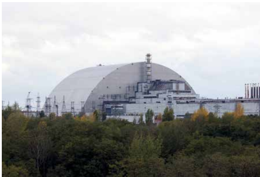
After the Chernobyl disaster, the reactor building was encased by a mammoth concrete sarcophagus which, in turn, has been supplemented by a “New Safe Confinement” in 2017.
