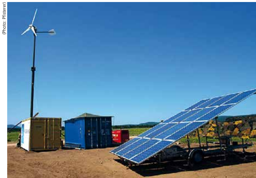
Photovoltaic modules, wind generator, and diesel generator build the core of a microgrid, as for example with the MEMS from Pfisterer.
