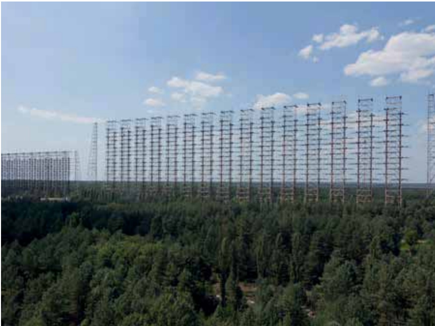
During the Cold War, Russia invested significant sums in OTH radar building the DUGA-1 (NATO reporting name Steel Work) system near the ill-fated Chernobyl nuclear plant in Ukraine.
