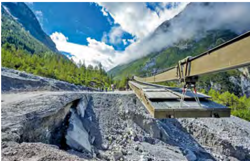
A WFEL Dry Support Bridge being launched over a landslide in Switzerland to allow the road to be rapidly reopened to civilian traffic
