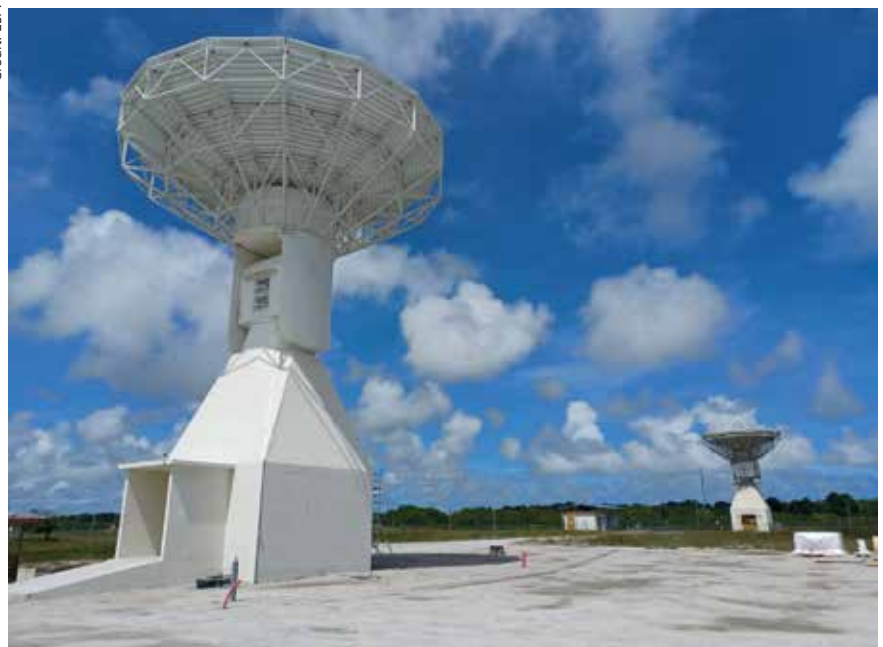
Galileo's new Telemetry, Tracking and Control (TT&C) facility is a 13.5 m diameter parabolic dish mounted on top of a 10 m structure. Known as TTCF-7, it is based at Kourou, French Guiana, beside the earlier TTCF-2.
