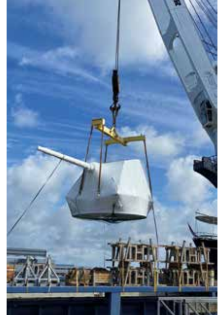
The Leonardo 127/64 LW Vulcano medium-calibre gun and associated ammunition handling system is being refitted to all ships of the De Zeven Provinciën class. HNLMS Evertsen is the first ship to receive the replacement gun
