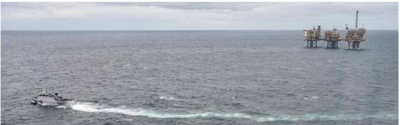
Oil and gas platforms are part of critical infrastructure in the North Sea. Targeting such infrastructure would be a non-kinetic, non-nuclear way for Russia to isolate NATO states.
